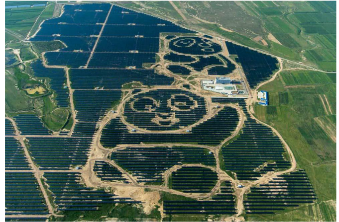
Fig. 18. Panda Power Plant. Source: GettyImages, utilized under Fair Use clause.
