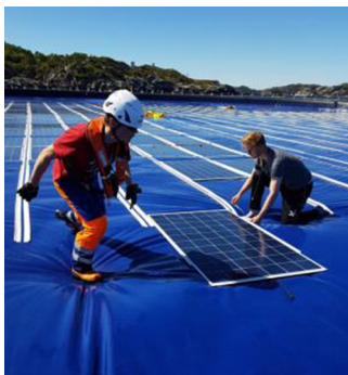
Fig. 4. Flat membrane design. Source: https://cleantechnica.com/2019/03/12/floating-solar-trampoline-by-ocean-sun-tested-by-statkraft/ .
