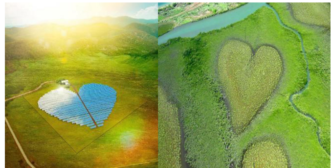
Fig. 19. Heart of Voh. Source: The Guardian. https://www.theguardian.com/environment/2014/sep/25/is-this-heart-shaped-solar-farm-the-worlds-most-beautiful-power-plant .
