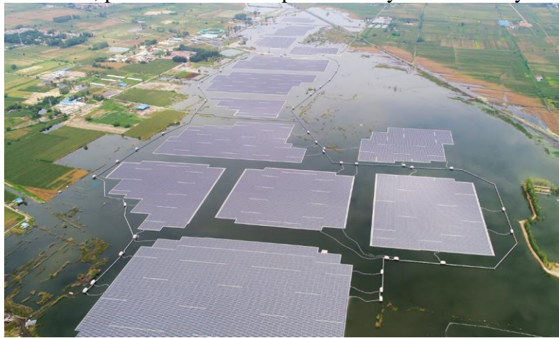
Ciel et Terre project in Anhui Province (Source: https://www.pv-magazine.com/2019/03/20/ciel-terre-completes-worlds-biggest-floating-pv-array-in-china/ )
